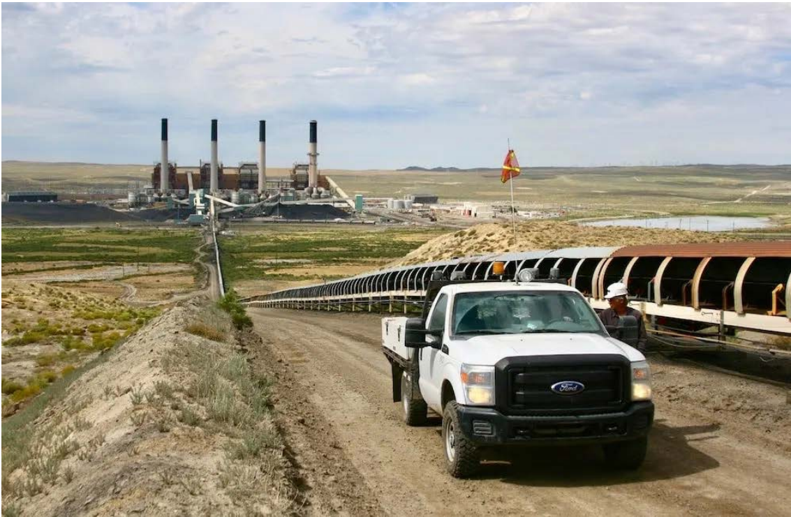
Figure 1: The Jim Bridger power plant
