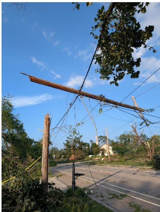
Snapped power pole after tornado in Appleton.
