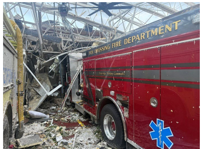
Apparatus damaged and fire station destroyed in Fox Crossing. Courtesy: Fox Crossing Fire Department.
