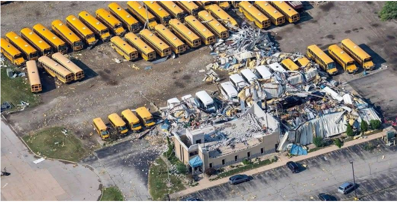
Damage to Lamers Bus Lines in Menasha.
