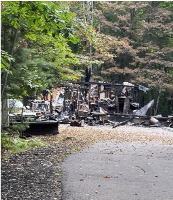
Home in Town of Washington in Vilas County was destroyed during July 27 storms.
