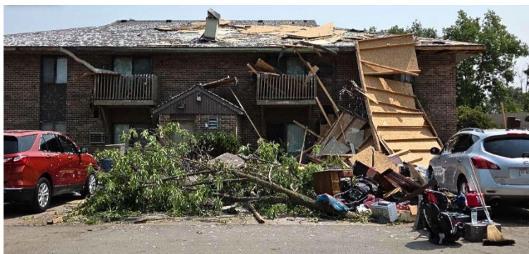
Grand Chute apartment building was damaged by tornado on July 27.
