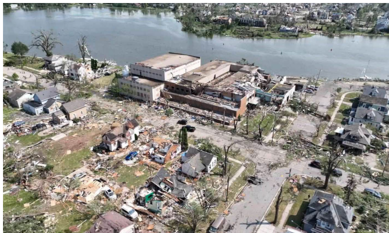
Damage to homes and City of Menasha Water Filtration Plant. Courtesy: WGBA.
