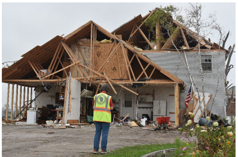
WEM staff conducting preliminary damage assessments.
