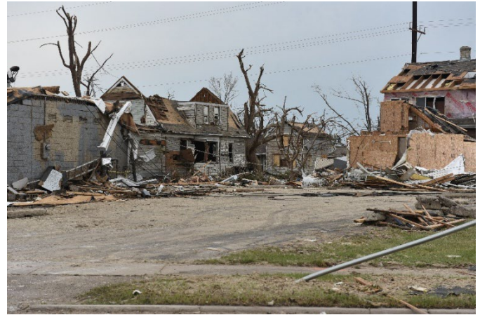
Several homes in Menasha were damaged after July 27 tornado.
