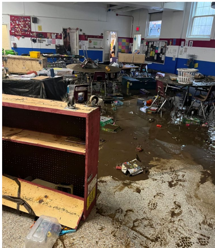
Photo: Flood damage inside Washington Elementary School in Janesville, WI. Courtesy: School District of Janesville
