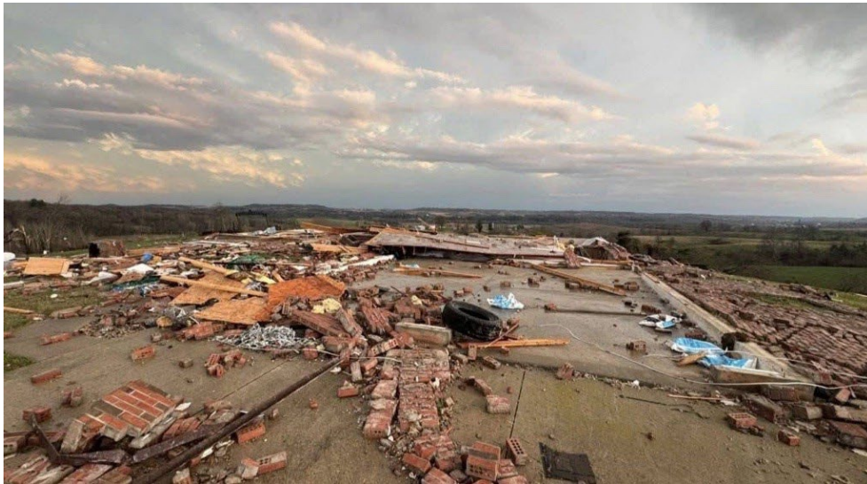
Photo: Home destroyed by tornado near Union Center, WI on April 14, 2026.
