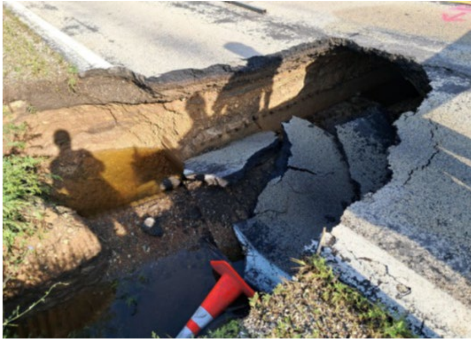
Photo: Culvert failure on City of Mequon road. Courtesy: City of Mequon Dept. of Public Works
