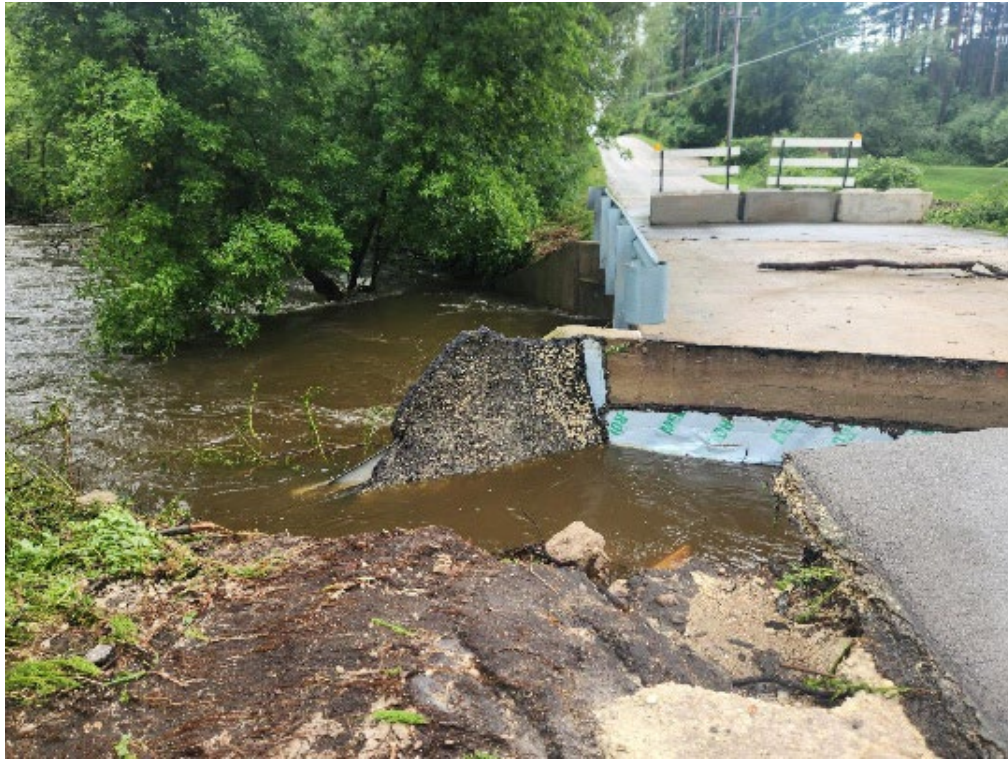
Photo: Flooding caused significant damage to the Indian Lore Bridge in the Town of Farmington, Washington County.
