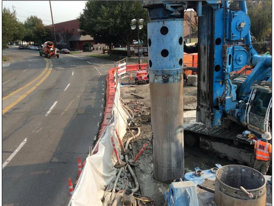
*The above photo shows secant pile wall construction currently underway at our Fremont site*
