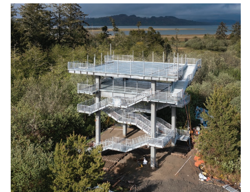
In 2021, the Shoalwater Bay Tribe partnered with Washington’s Emergency Management Division and FEMA to construct a tsunami evacuation tower to keep the community safe in the event of earthquake and tsunami.
