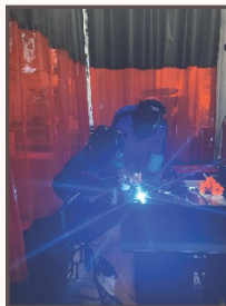
Haley applying the initial tack welds to the frame
