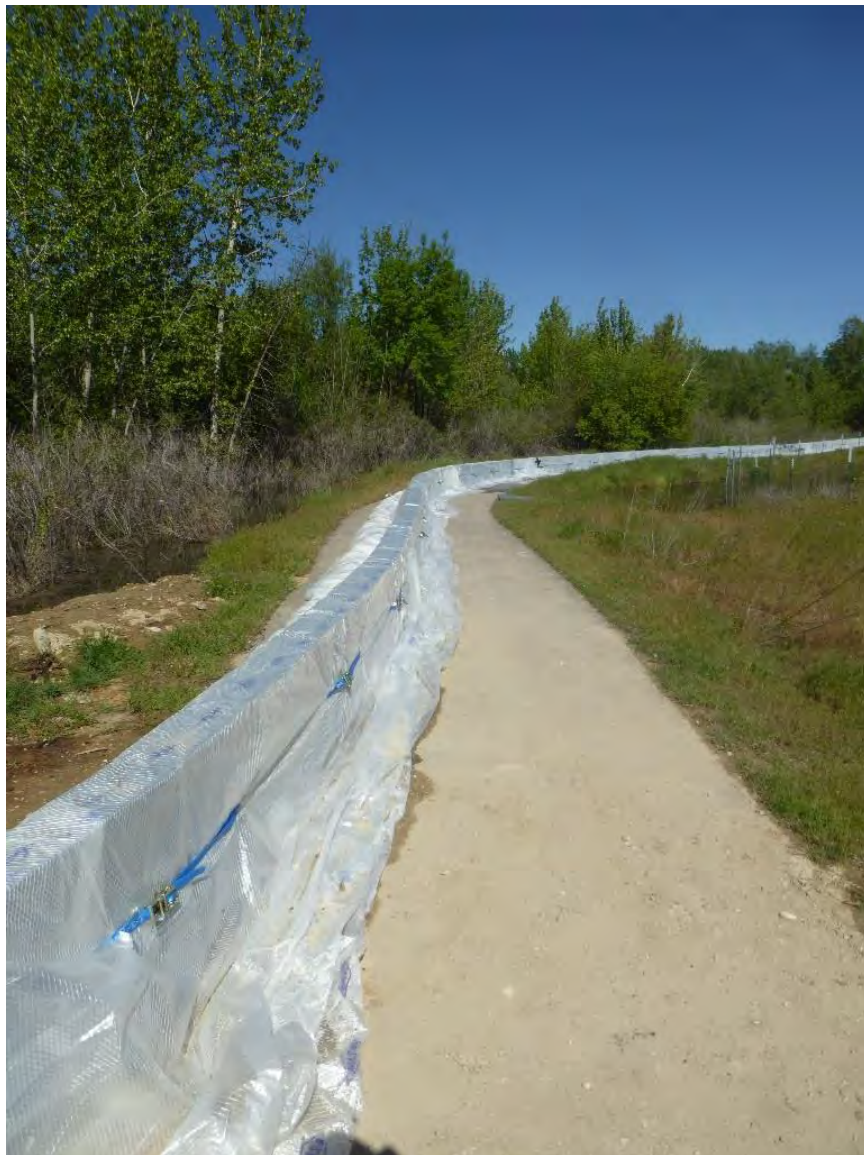
Figure 9. Muscle Wall Flood Barrier Deployed on the Boise River, Idaho, 2017.
