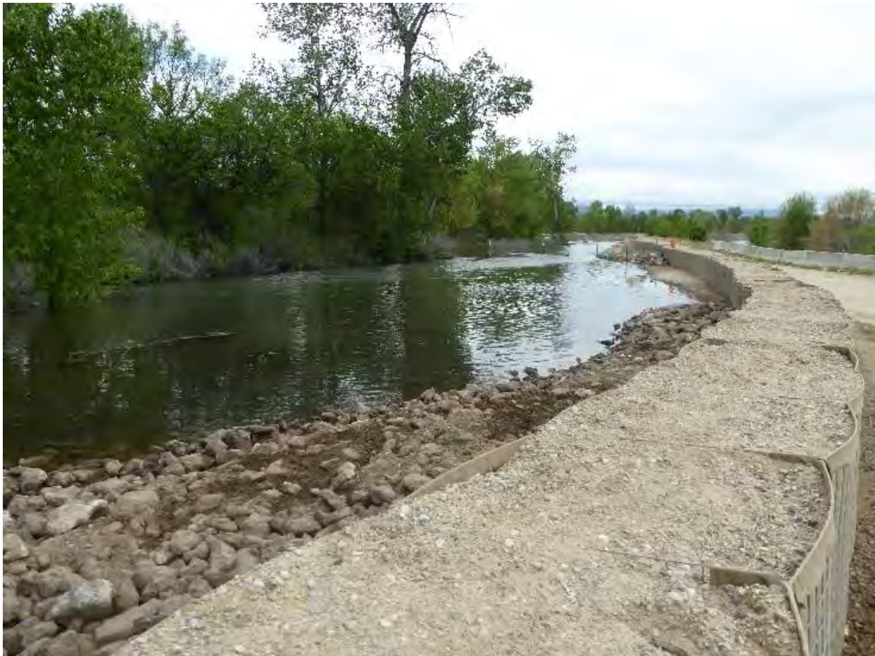
Figure 8. HESCO Barriers Deployed on the Boise River, Idaho, 2017.
