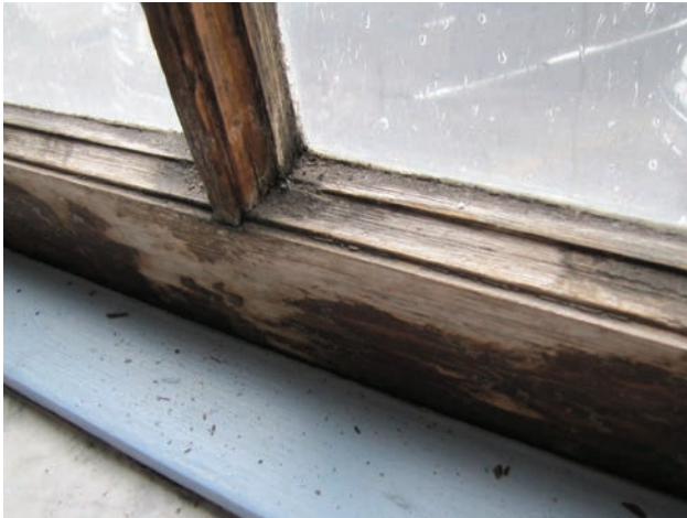
Window sash damage due to uncontrolled condensation.
