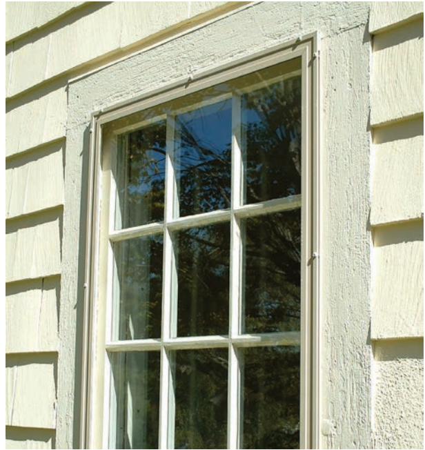
A more compatible exterior metal storm window, as compared with previous image.
