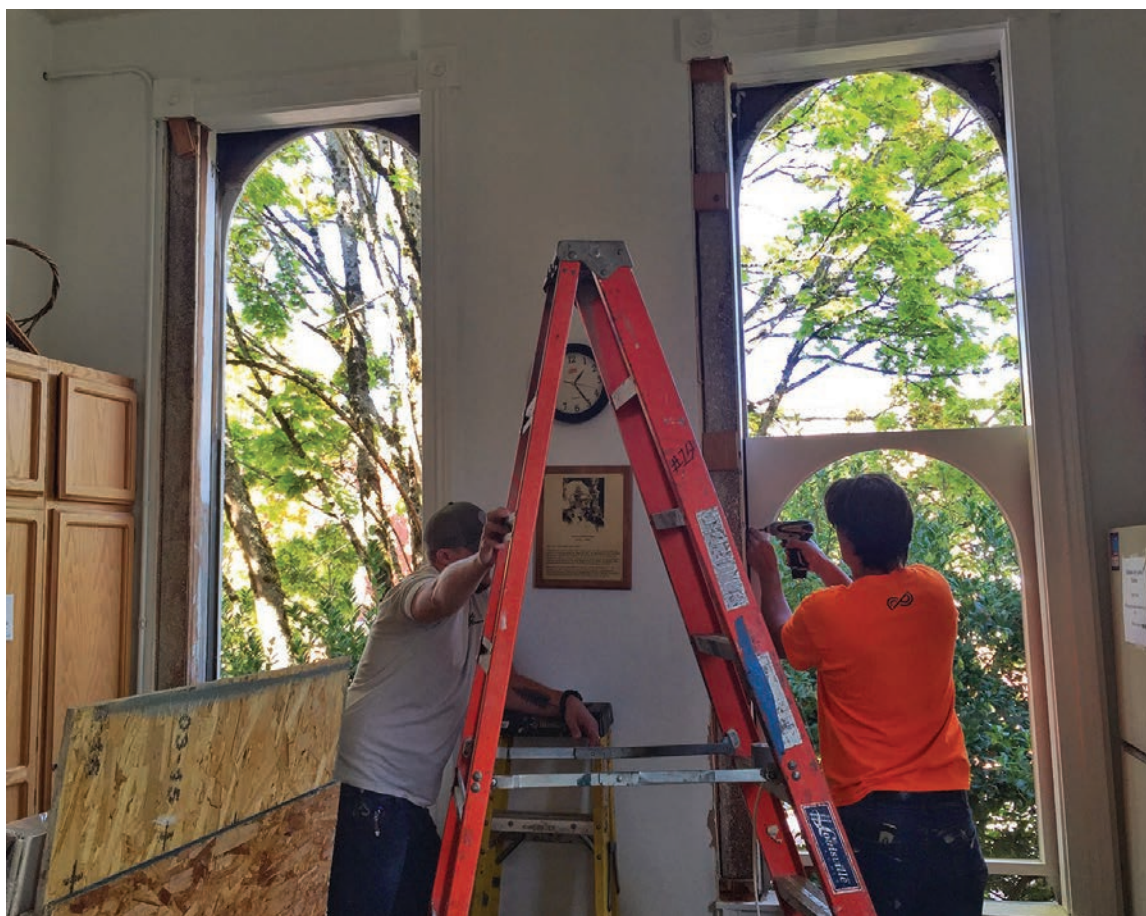
Workers removing historic windows for transport to their workshop.
