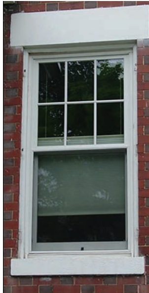
Replacement window designed to be installed within the jamb. It represents about the best that can be accomplished in this way.
