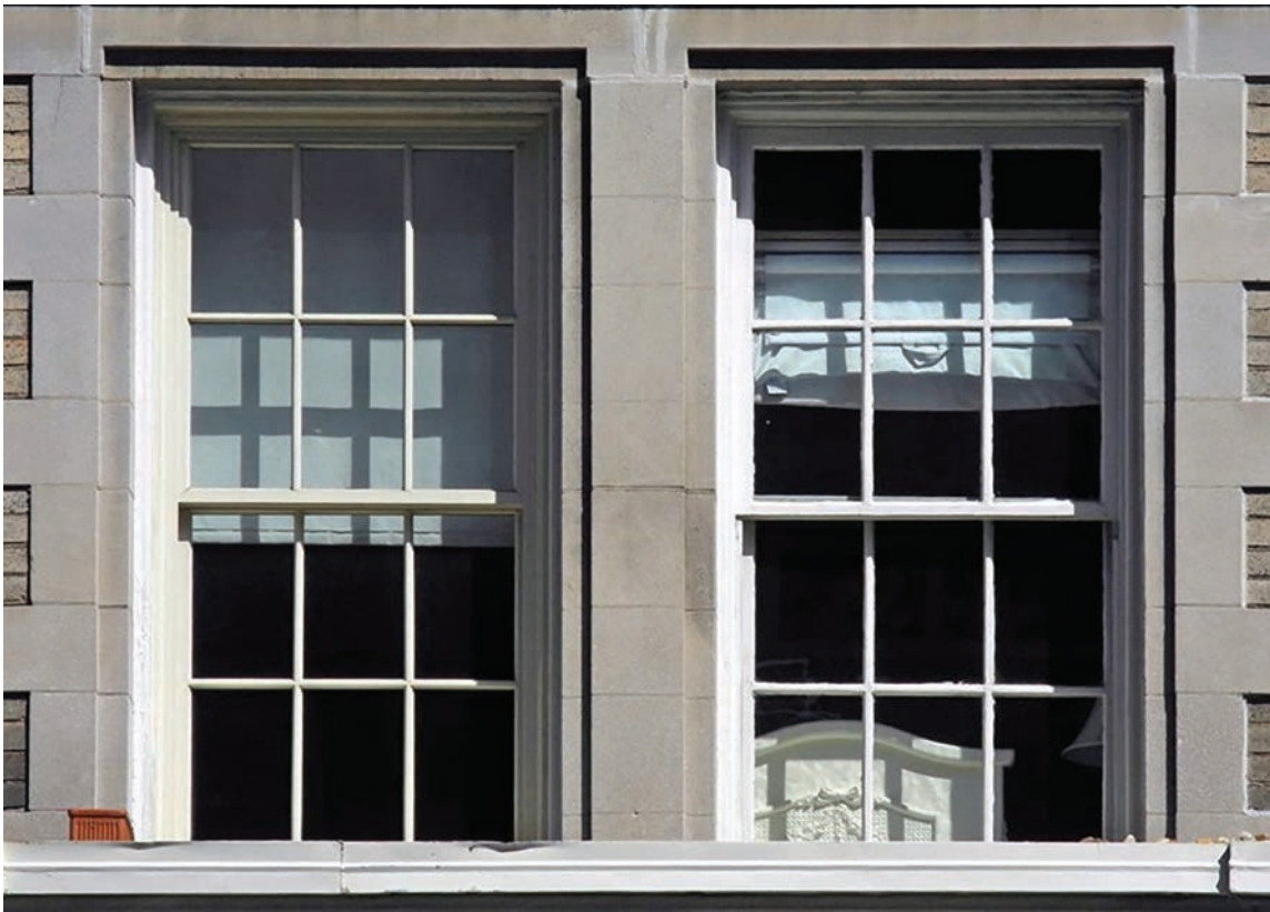
An example showing an original window on the right, with the replacement on the left. You can see just how the left replacement is different, but how it may not matter at a normal viewing distance.
