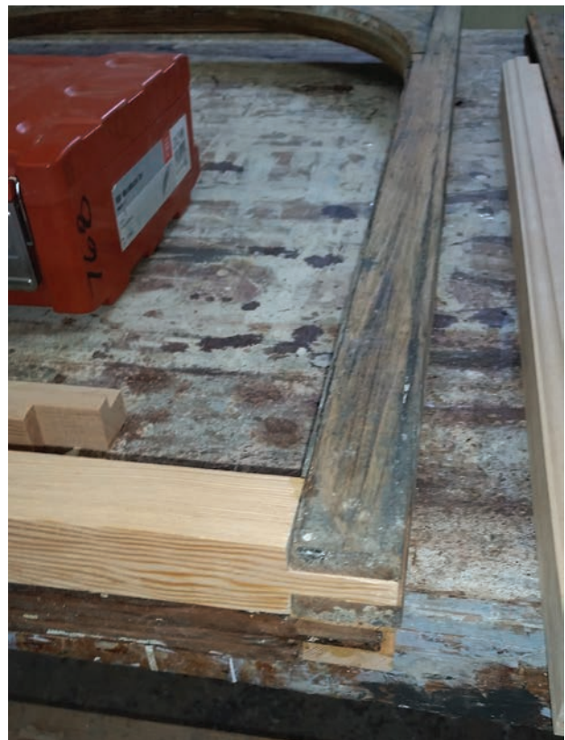
Installing new components to historic wood window.
