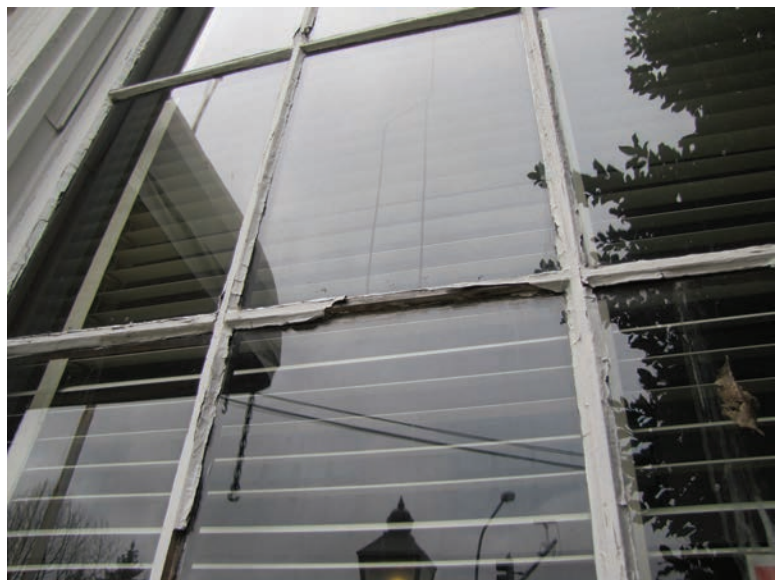
Multi-light wood window that just needs to be re-puttied and painted
