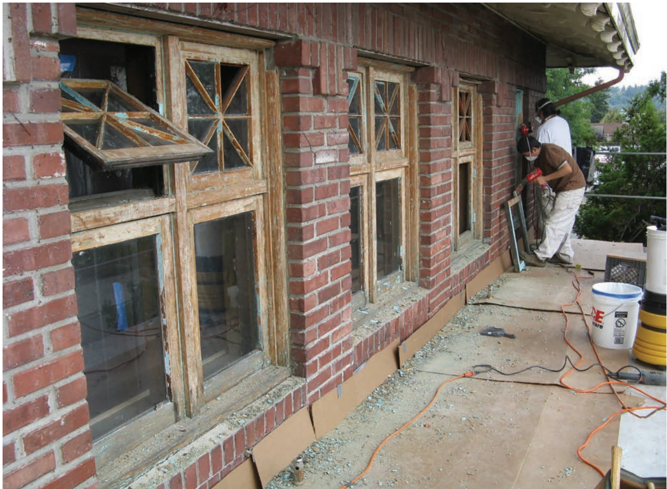
Decorative pivot windows being re-puttied and painted in place.
