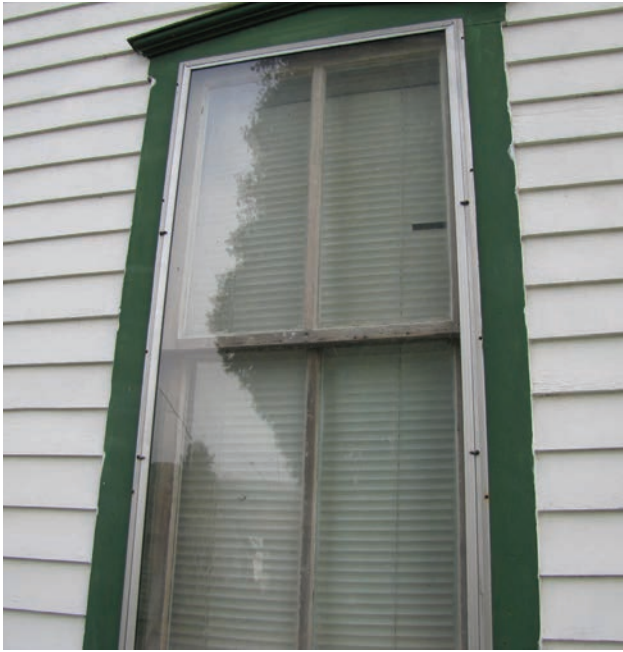
A less compatible exterior metal storm window, as compared with next image.
