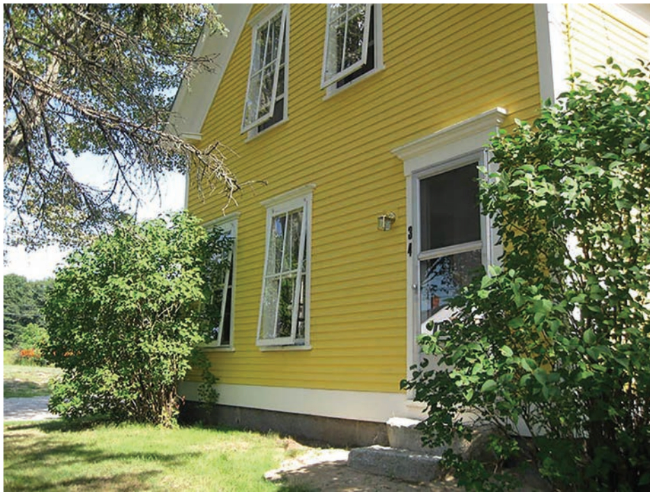
Exterior wood storms, opened to provide ventilation.
