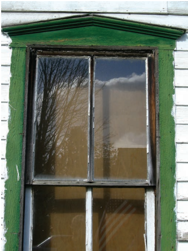
A circa 1905 double hung 2/2 wood window in need of some TLC.
