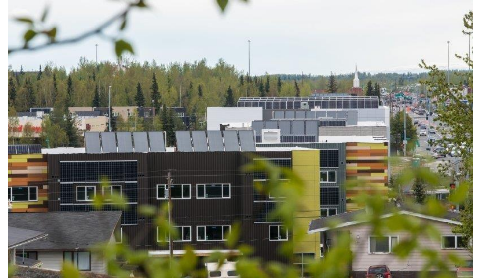
Residential solar project in Anchorage, Alaska (Source: DOE, EERE)
