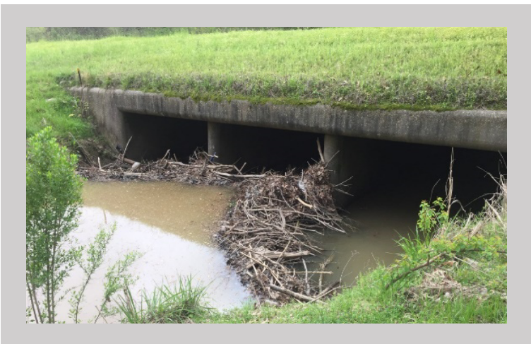
Figure 1. Photo credit: USFS. The damming of box culverts is a typical example of the problem that will be addressed with the technologies presented during the webinar.
