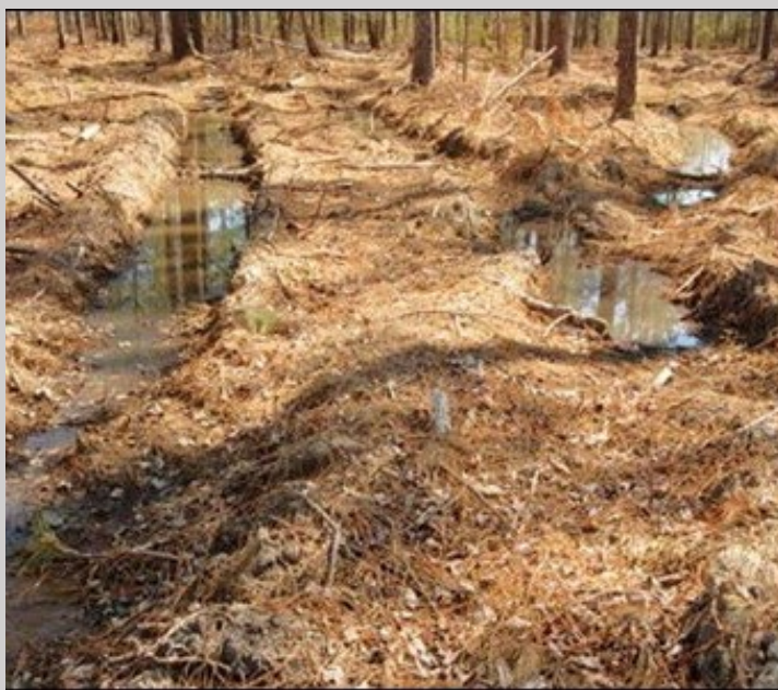
Figure 1. Photo credit: USFS. The rutting on this native surface road is an example of a problem that will be addressed with the technologies presented during the webinar.
