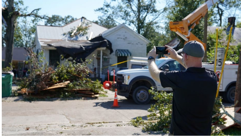
Figure 1. Taking photos of a damaged home after a disaster event
