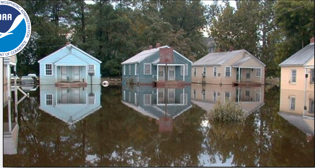
Downtown Franklin, VA inundated by flood waters Photo credit: FEMA
