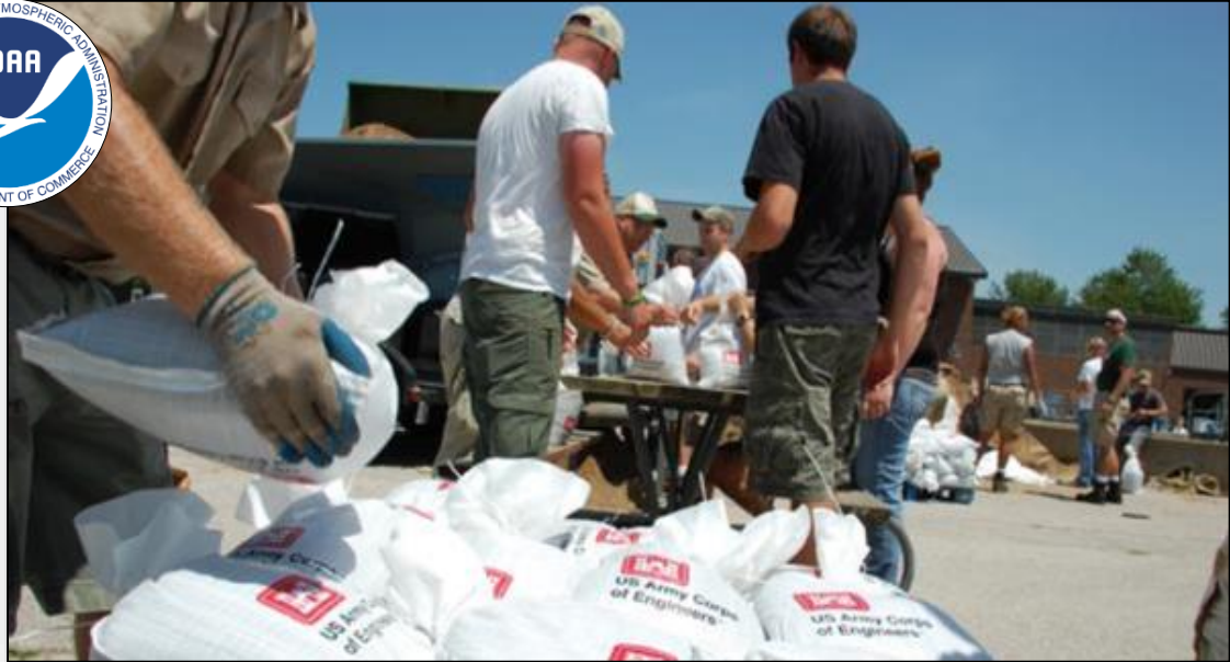
Volunteers prepping sandbags ahead of expected flooding along the Chariton River in IA Photo credit: FEMA
