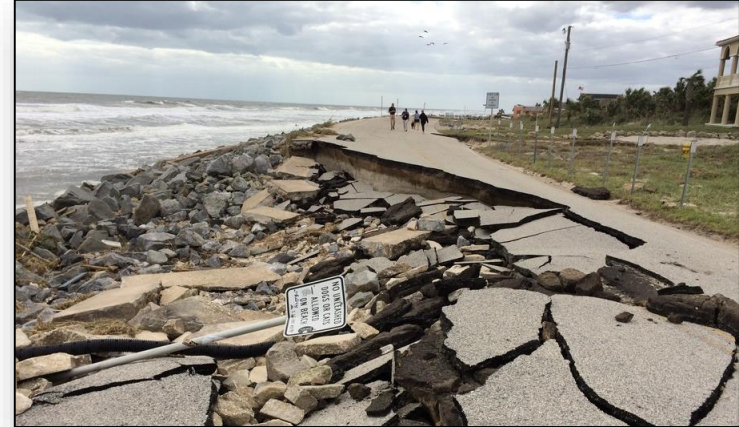
FEMA Officials Survey Damage on Highway A1A near St Johns county Photo Credit: Eileen Lainez
