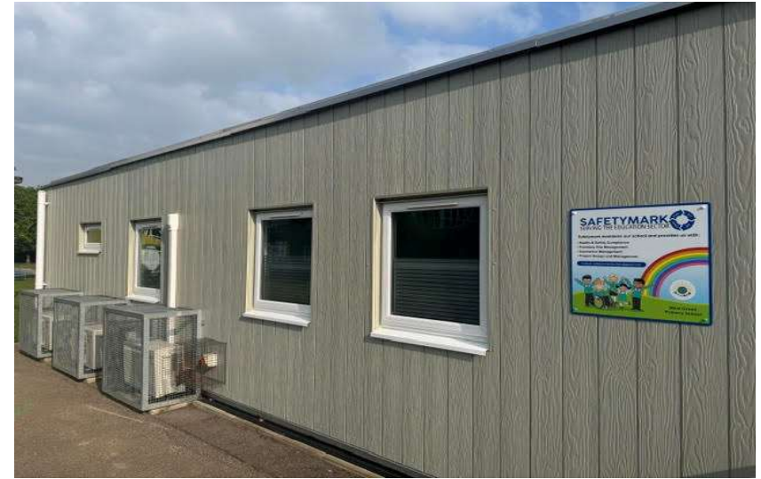
New air conditioning/heating units Whole building with cedar cladding
