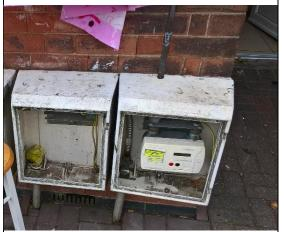
The utility boxes at the property were damaged and did not have locking doors for security and safety.
