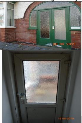
There is HHSRS hazards of collision and entrapment and excess cold at this property as it is not fitted with safety glass in the critical location of the entry door and it is single glazed to a large area. The glazing leaves the property lacking in adequate security measures with the poor quality doors and windows with no security lighting.
