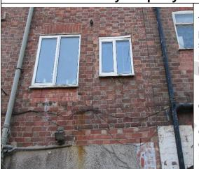
The exterior of the property was in poor visual condition, as per example 6 above, this can include trailing cables, disused satellite, broken aerials or other defective and redundant installations and signage. The window is propped open with a plank of wood.
