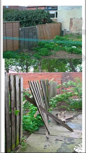
The garden wall and fence look to have been repaired but remain defective and require repair. The exterior wall of the property is a miss match of colours and looks poorly maintained.
