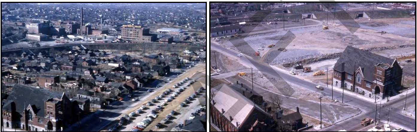
Figure 5. Photographs of the Capitol Hill urban renewal project along Charlotte Avenue, 1956. The right image shows the St. John's AME Church (right), demolished in 1957, and First Baptist Church, Capitol Hill (lower left). Scores of dwellings were demolished for state employee parking lots and James Robertson Parkway (Source: Tennessee State Library and Archives).
