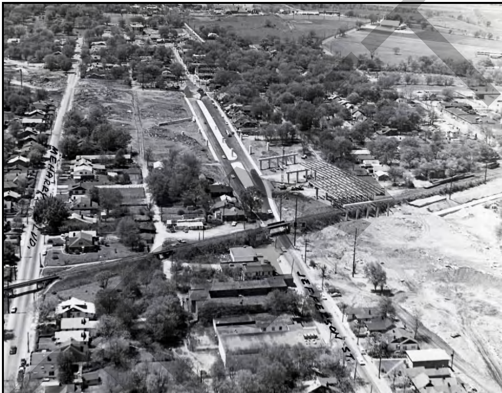
Figure 31. Aerial photograph of the I-40 overpass and interchange with Jefferson Street under construction, circa 1969 (Source: Nashville Public Library Special Collections).
