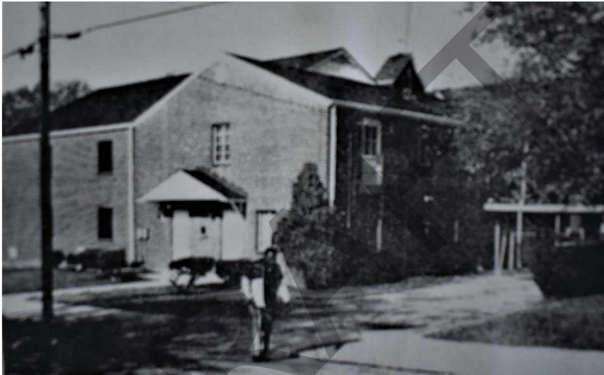
Figure 15. Photograph showing the 1981 wing (far left) under construction, looking northwest (Source: Clark Memorial United Methodist Church Archives).
