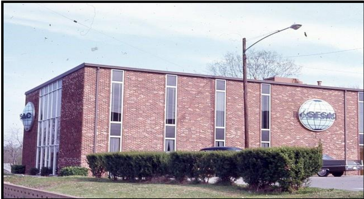
Figure 20. SESAC opened a modern-style office building in 1970 at 11 Music Circle South (DV.26105) on Music Row. Source: Metro Nashville Archives.
