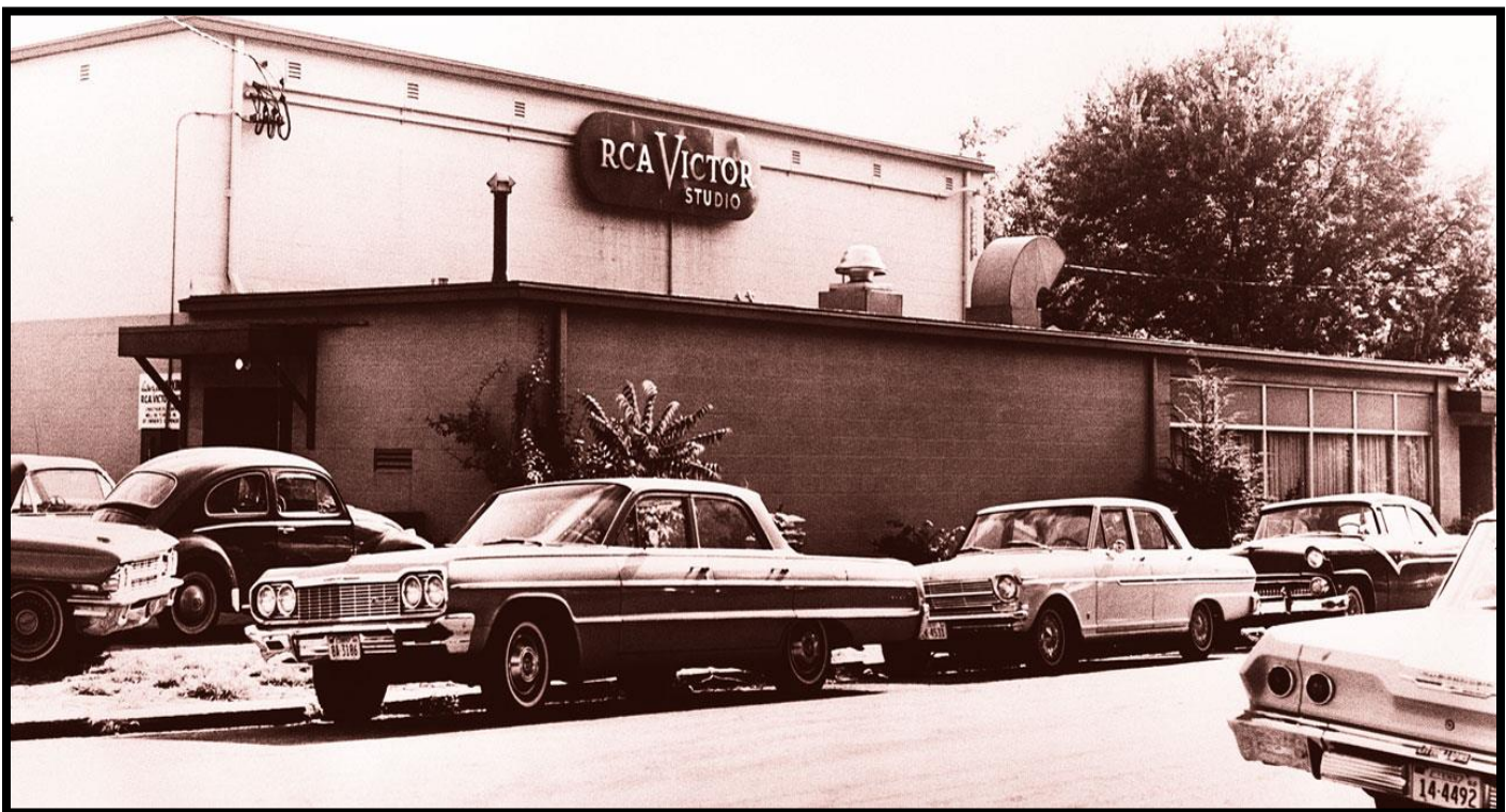
Figure 6. RCA Studio B (DV.26100), circa 1962, built in 1957 at the corner of 17 th Avenue South and Hawkins Street (now Roy Acuff Place). Source: Country Music Hall of Fame and Museum .
