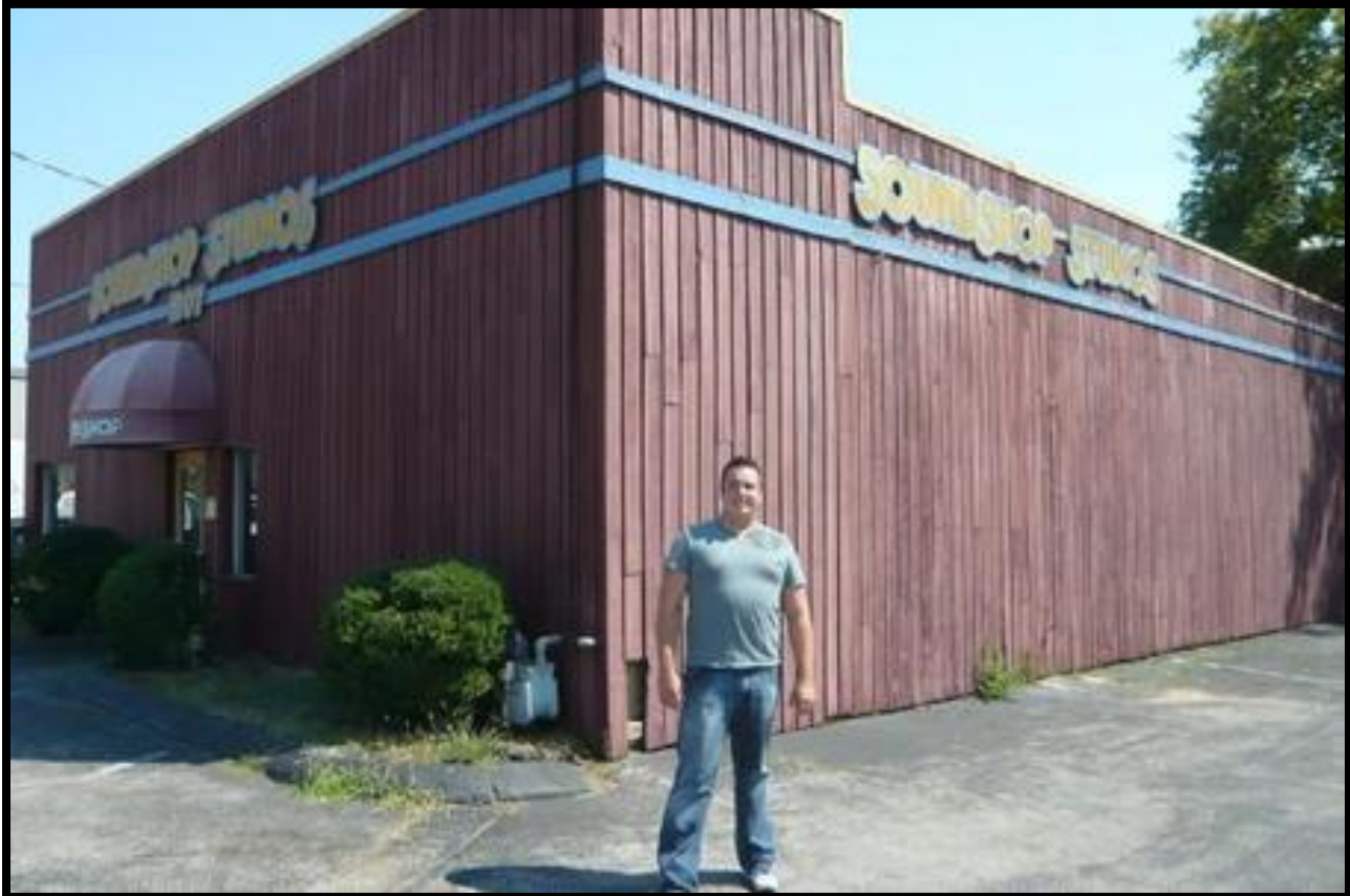
Figure 14. Sound Shop Studios on Division Street, undated. Demolished January 2015. Source: Coy Taylor.
