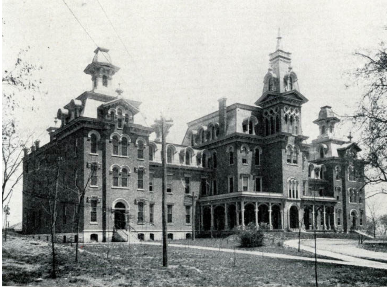
TENNESSEE SCHOOL FOR THE BLIND.
