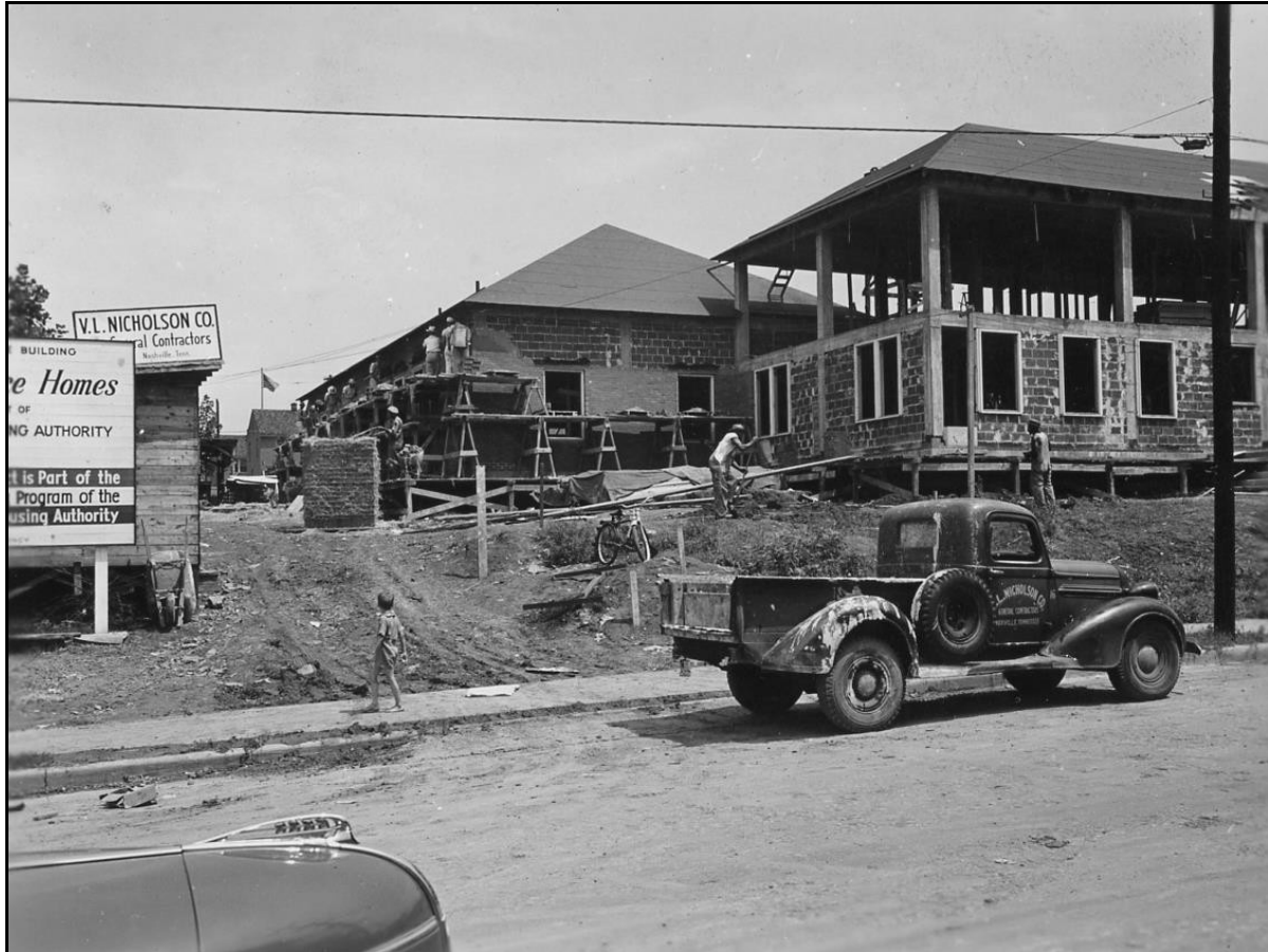
Figure 1. Construction of the James A. Cayce Administration Service Building in 1942. (Metro Nashville Archives)
