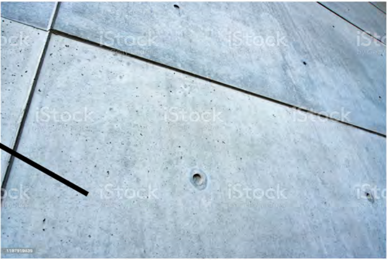
CAST IN PLACE CONCRETE
