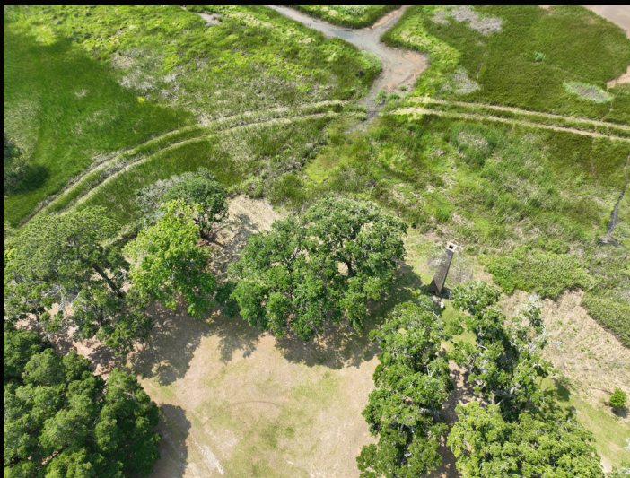
Figure 1. Aerial photograph of rice mill chimney and former rice fields. Photo by Kendy Altizer.
