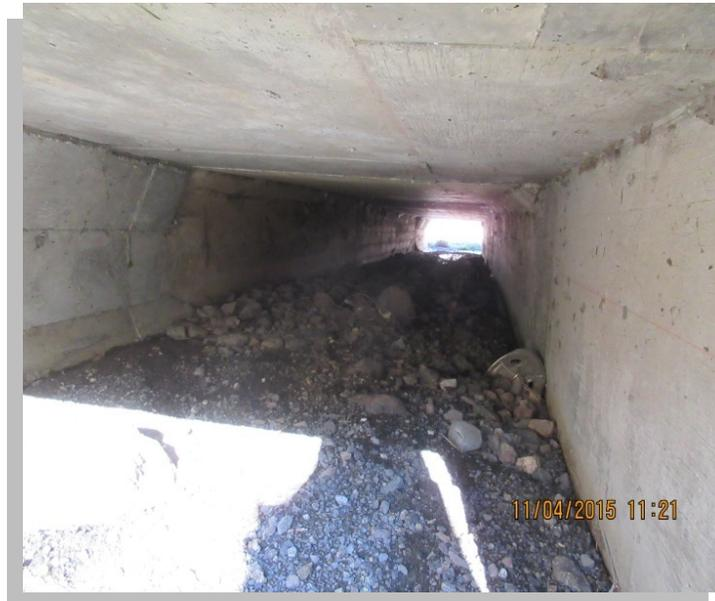
The existing culvert does not meet current fish passage criteria.
