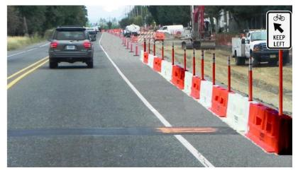
lightweight plastic barrier system that guides cyclists along a pathway, keeping them from entering into active work areas or coming into contact with workers or equipment. Development of additional design standards and application details are currently underway. ODOT is expecting to use a bicycle channelizing device in a highway construction starting in June 2016.
