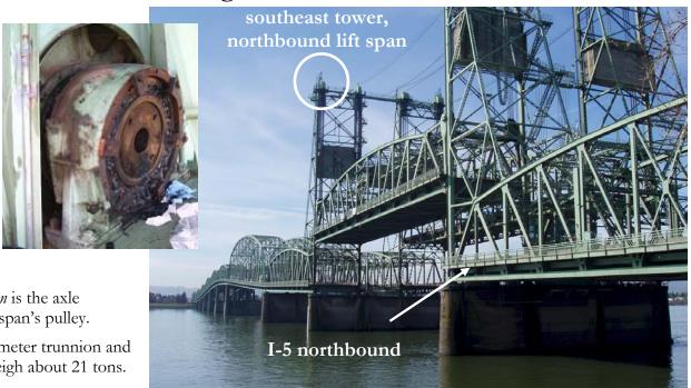
A *trunnion* is the axle of the lift span's pulley.
