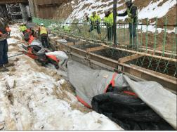
After completing the northern half, crews continue excavation, pile driving, and pouring footings for the southern half of the Knox Avenue Transitway. As part of the METRO Orange Line, the tunnel connects Bloomington and Richfield via I-35W underneath I-494. Its entrance is near the Knox Avenue Park & Ride by Best Buy headquarters in Richfield. The transitway will also include a bike path. The Orange Line is scheduled to begin service in late 2021.
