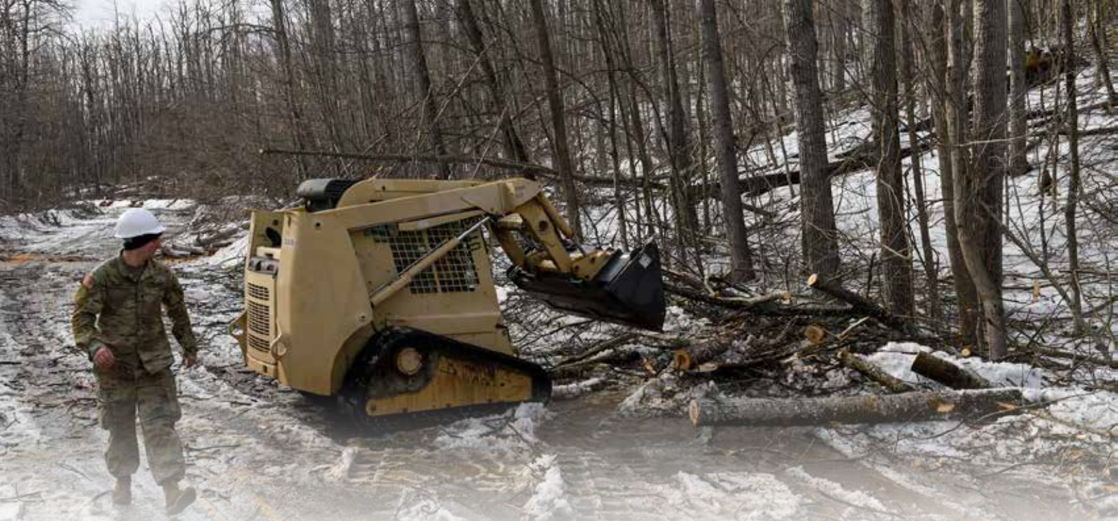
Sgt. Marcus Martin, assigned to the 1434th Engineer Company, 107th Engineer Battalion, 177th Military Police Brigade, Michigan National Guard, operates a skid steer to clear debris from a roadway following a severe storm outside Alanson, Mich., April 3, 2025. (U.S. Army National Guard photo by Daniel Garas)
