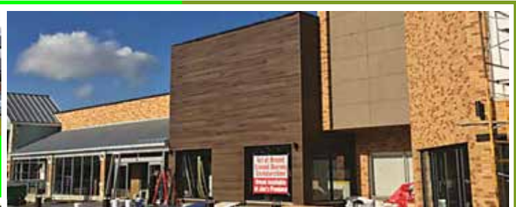
Joe's exterior facade renovations bring a completely new look to the shopping center
