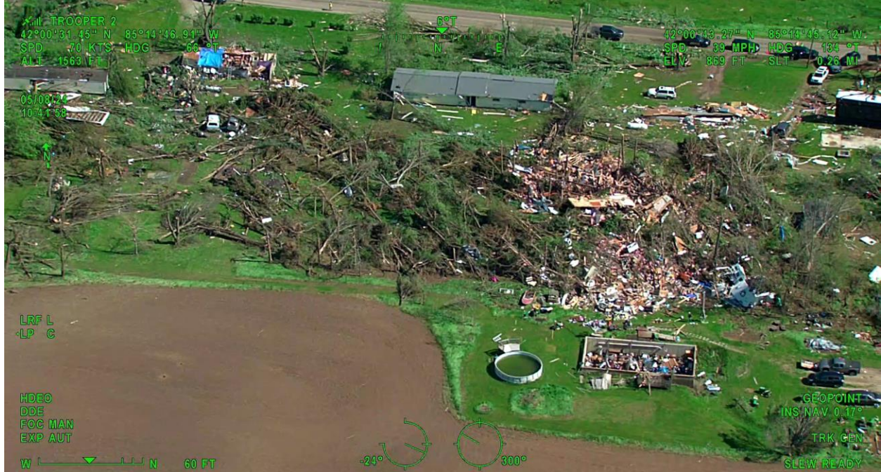
Image 1: Tornado damage in Sherwood, MI. Photo courtesy of MSP Helicopter Survey.
