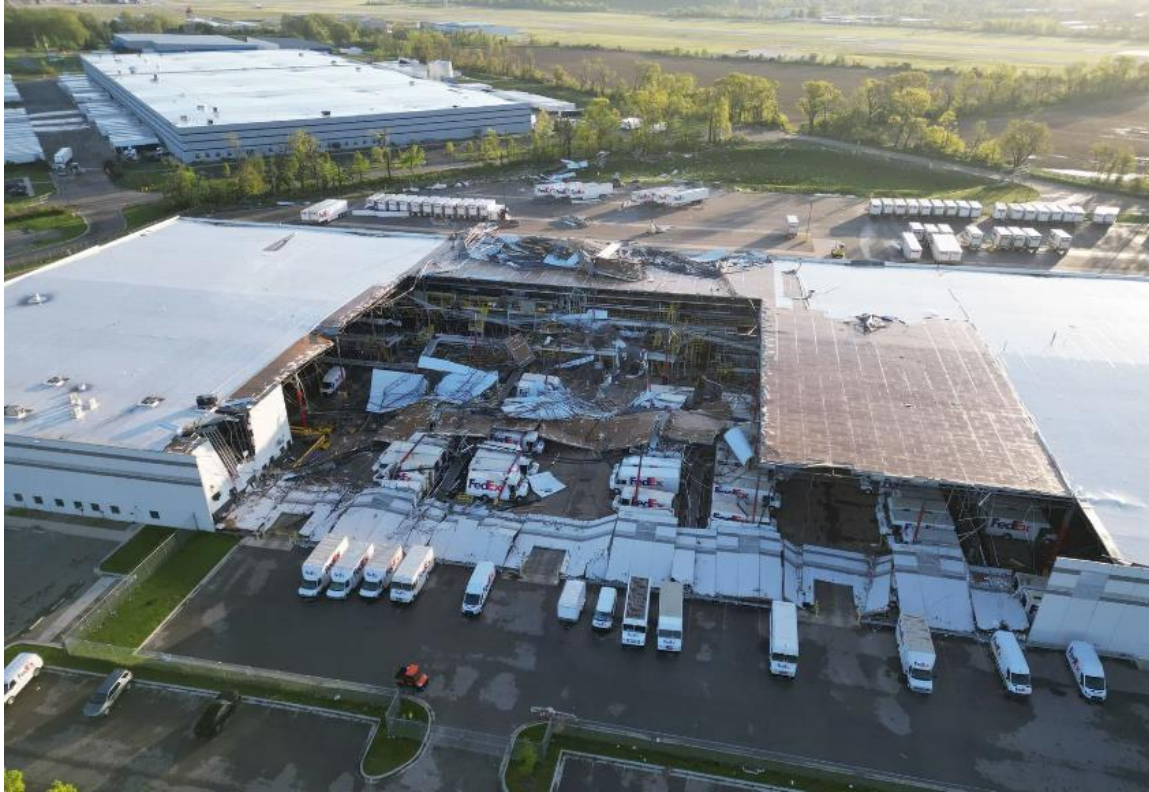
Image 5: Roof damage to the FedEx facility in Portage, MI (Kalamazoo County tornado). Photo courtesy of Jake Taylor/WWMT.
