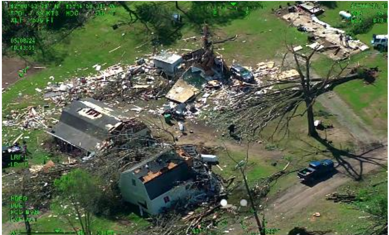
Image 2: Tornado damage in Sherwood, MI. Photo courtesy of MSP Helicopter Survey.
