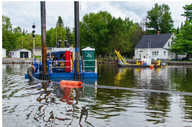
A contractor working for the U.S. Army Corps of Engineers dredging the Grand Traverse Harbor in August 2019. (Michigan DNR photo)
