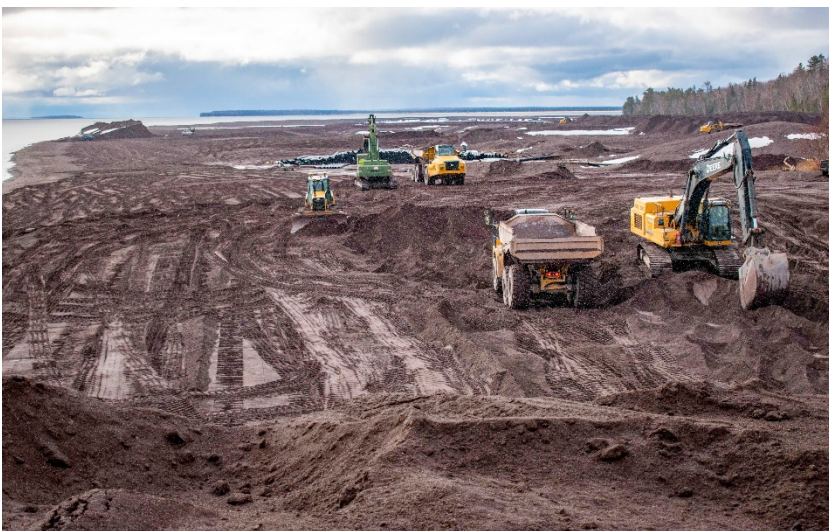
A 30-foot-high bank of stamp sand deposits is being removed from the Lake Superior shoreline at Gay in November 2019. (Michigan DNR photo)
