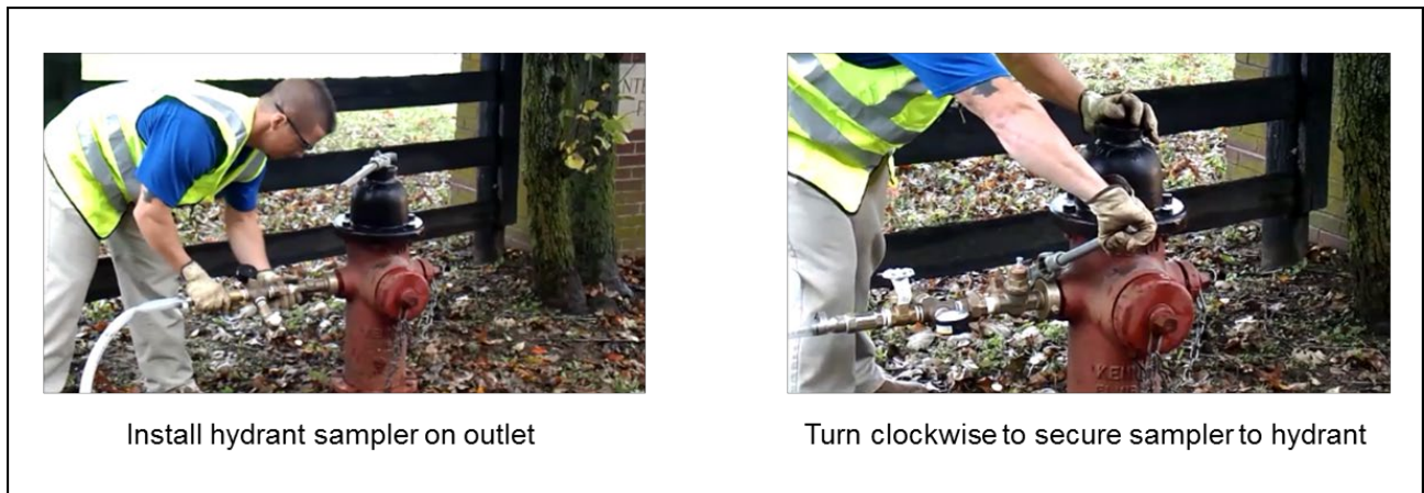
Figure 4. Install hydrant sampler on hydrant
