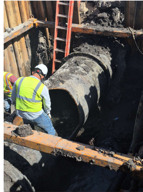
Tuesday February 24 th Repairs underway; BWA cancelled*
