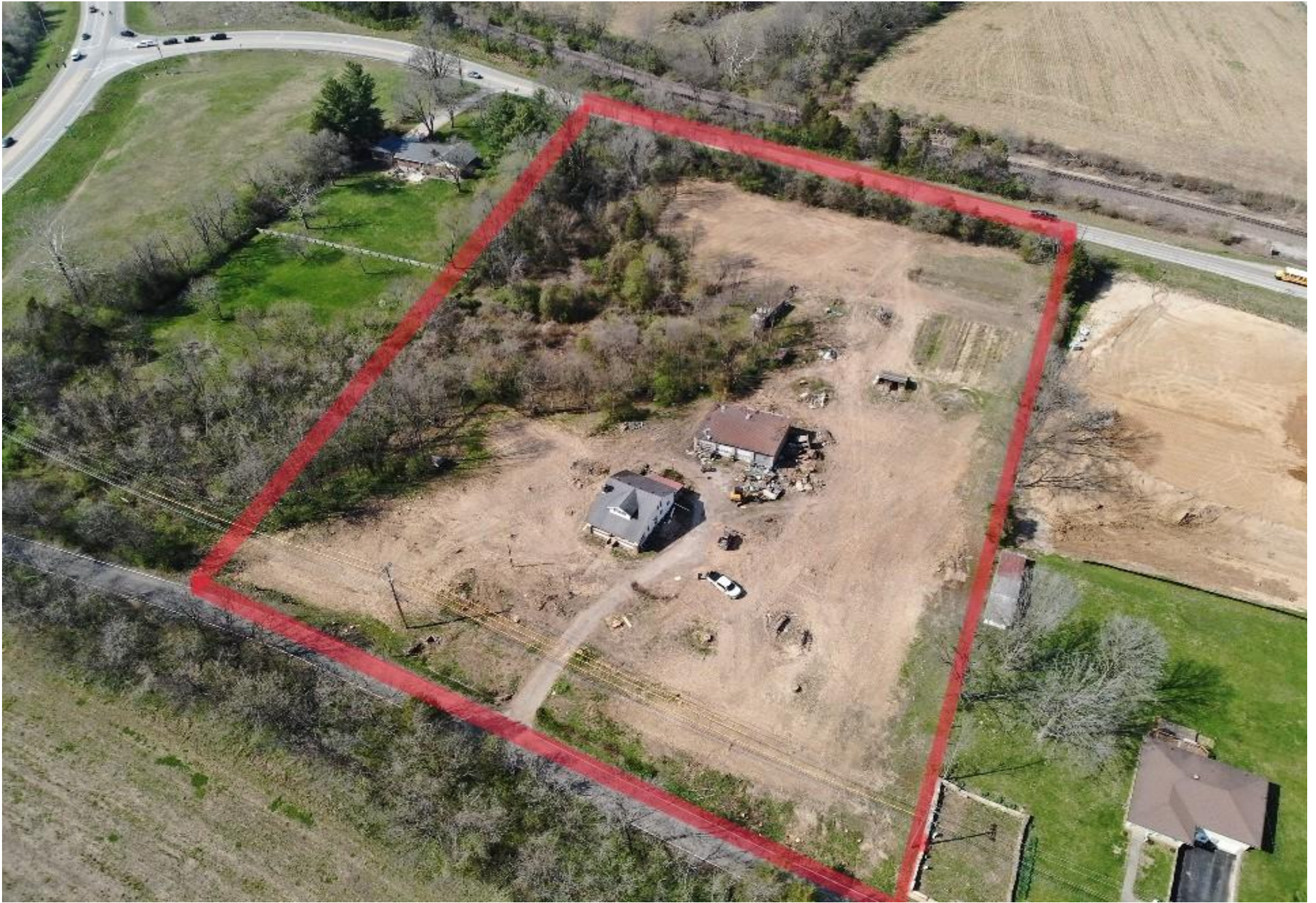
This image shows approximate property boundaries and final necessary land clearing.
