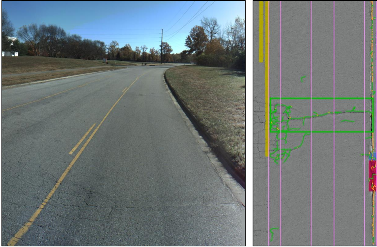
Figure 5.2.2.a: Mandli Right of way (ROW) imagery of a road with a PCI score of 58 , which is on the lower side of Fair (Left). Figure 5.2.2.b: Image of the LCMS RAGE Downward Image with Overlay of the road depicted in Figure 5.2.2.a.
