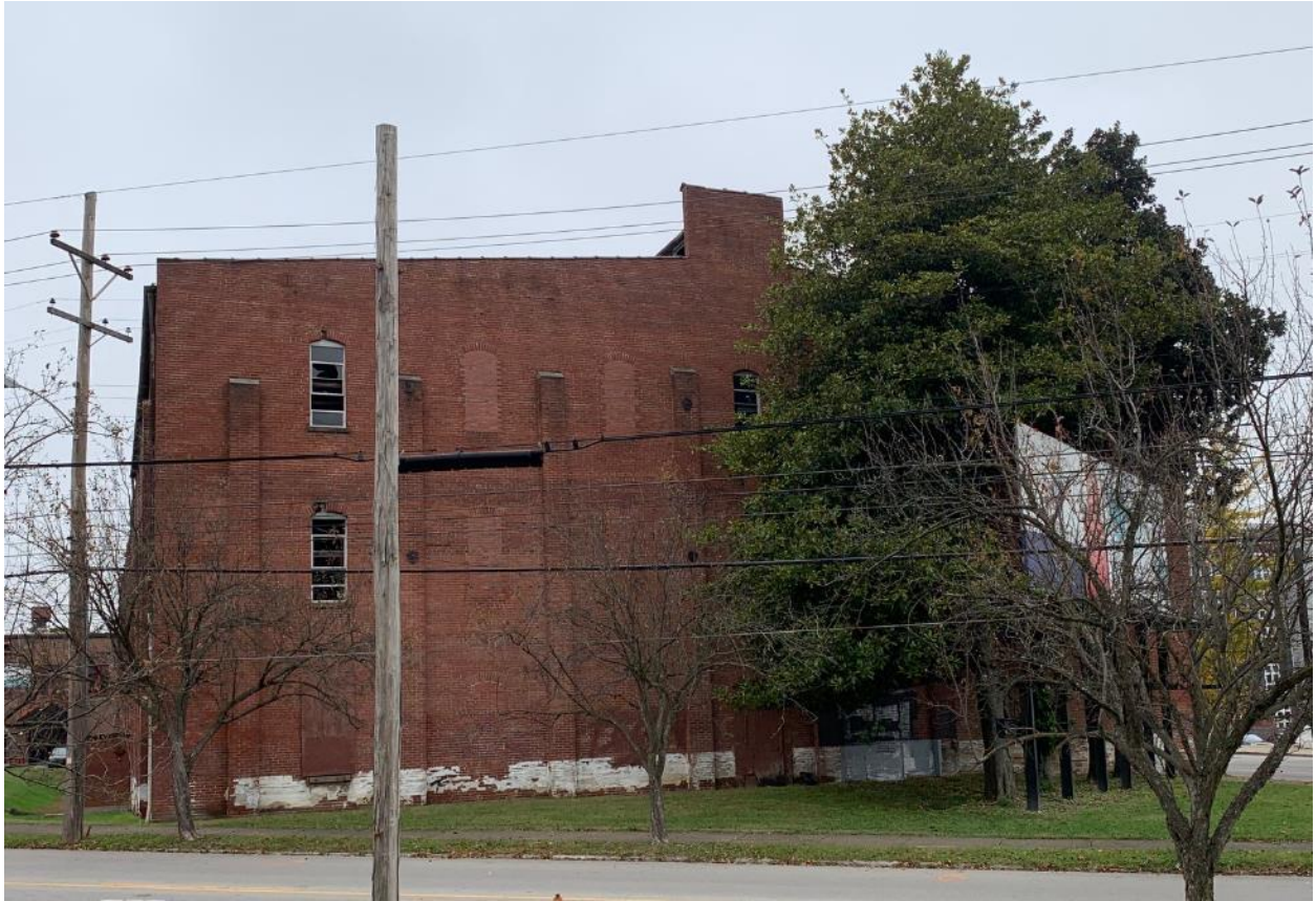
East Elevation (Staff Photo October 2020)
