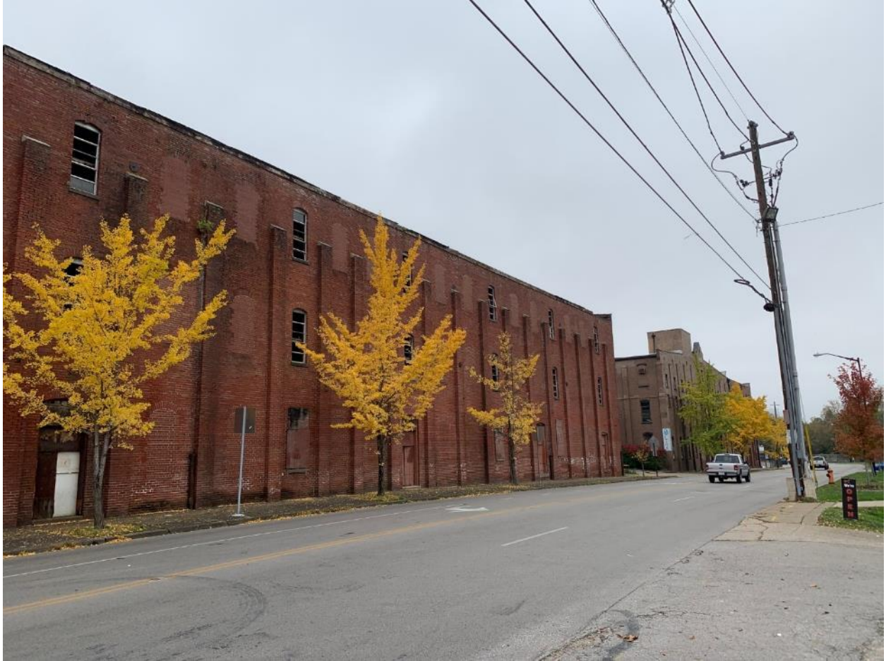
North Elevation (Staff Photo October 2020)
