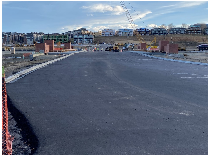
Marshall Road Bridge Paving
