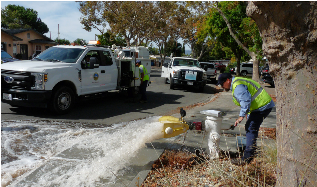
Flushing water mains provides the highest water quality possible.
