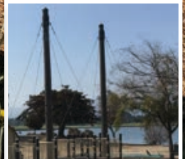
Shoreline Play Structure Replacement Construction in fall 2025
