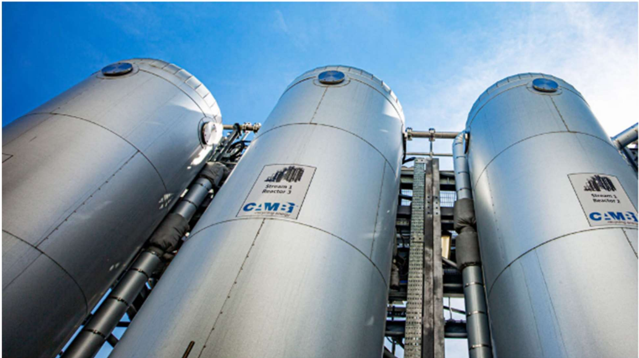
The Cambi thermal hydrolysis process (THP) was installed to preheat and jumpstart the breakdown of wastewater solids. Pressurized THP reactors above.
