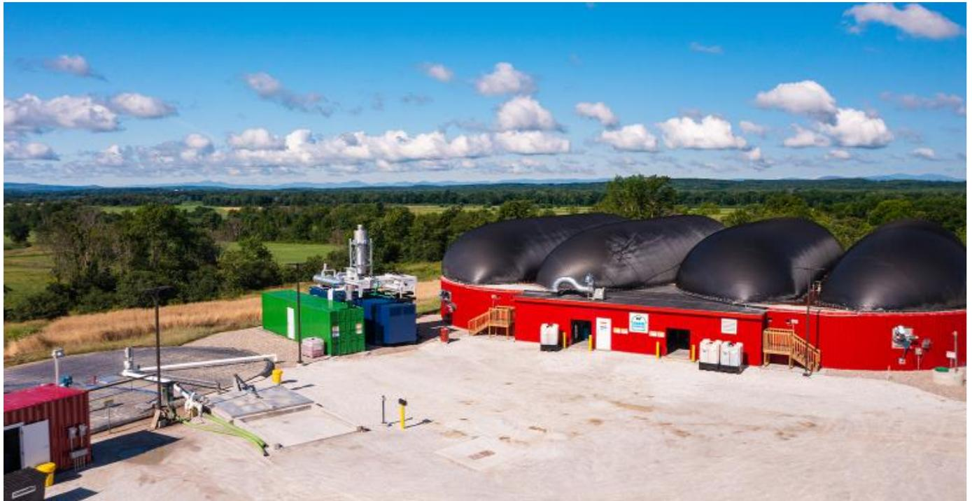
A Vermont farm, neighboring college, and utility are partnering with Vanguard Renewables on a project that has capacity to convert about 180 tons of food and beverage waste and 100 tons of manure into renewable natural gas (RNG) each day. The anaerobic digestion (AD) operation, reportedly the largest in New England, comes with advantages unique to each party's interests, while giving Vermont food producers an outlet for mega volumes of scraps.
