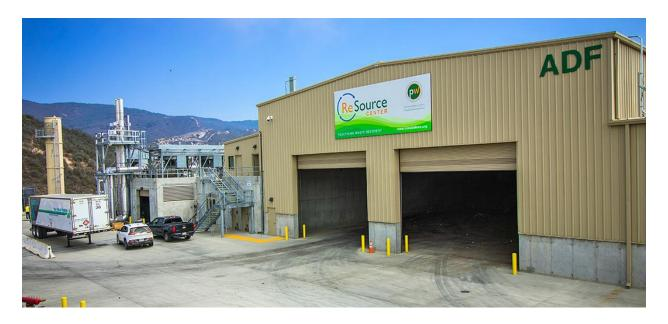
The first scoop of sorted organics from the southern part of Santa Barbara County, California was loaded into a bunker at the county's Anaerobic Digester Facility (ADF) in late August. The facility's design capacity is 74,600 tons/year. The county selected a Bekon dry fermentation system. This is the first U.S. installation for Bekon, which is based in Germany.
