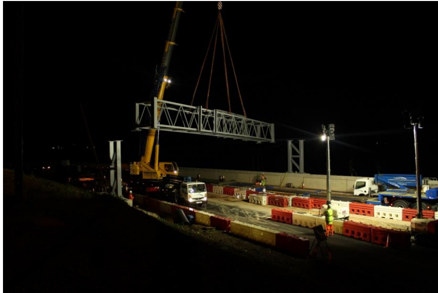
Photo 3: Gantry 21A installation across the mainline dual carriageway.
