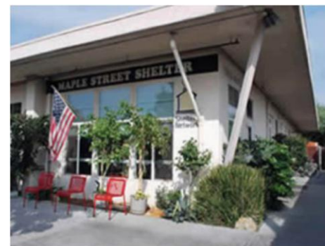
Maple Street Shelter, Redwood City, CA
