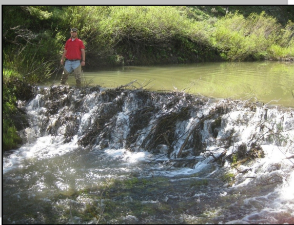
One of the beaver dams present on Bare Creek.
