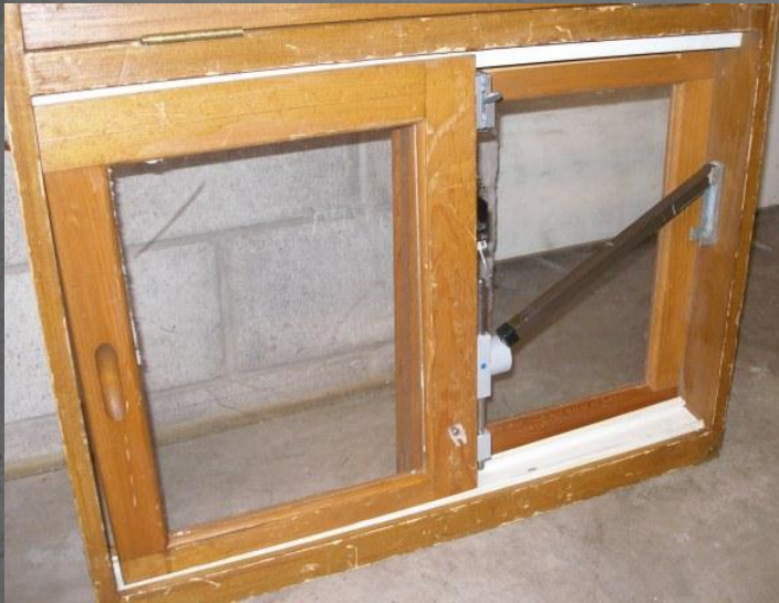
Sliding window closed, locked. Charley bar and other locks shown.
