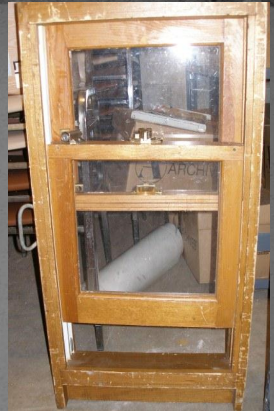
Pinned double hung window opened 6" for ventilation. This is secure.
