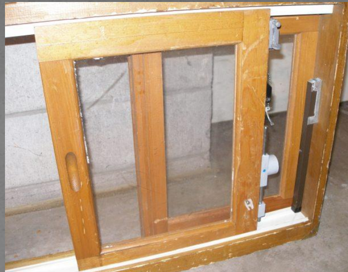
Pinned sliding window opened 6" for ventilation. This is secure.
