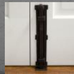
Example of a surface bolt.
