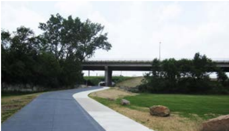
Phase 3 - East of I35W Tunnel
