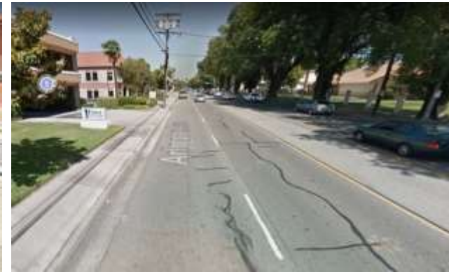
Arlington Ave - Indiana Ave to Magnolia Ave (Bike Lane)
