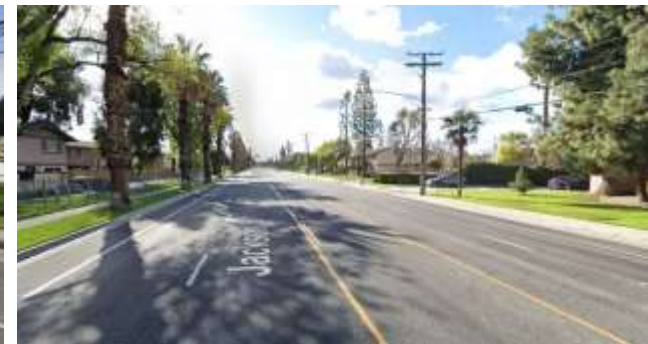
Jackson St – Van Buren Blvd to Colorado Ave (Bike Lane)
