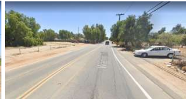
Washington St - Victoria Ave to Van Buren Blvd (Bike Lane)
