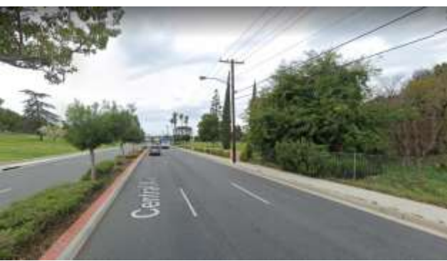
Central Ave - Victoria Ave to Brockton Ave (Bike Lane)
