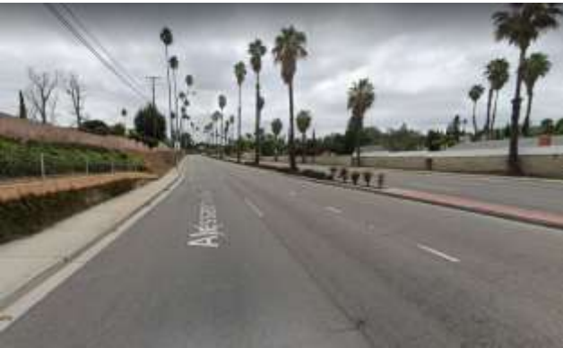
Alessandro Blvd- Chicago Ave to I-215 (Buffered Bike Lane)
