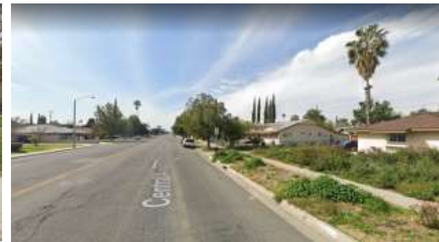
Central Ave - Hillside Ave to Streeter Ave (Buffered Bike Lane)
