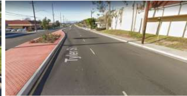
Tyler St - Wells Ave to Arlington Ave (Bike Lane)
