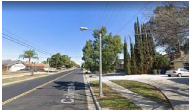
Colorado Ave - Jackson St to Adams Ave (Bike Boulevard)
