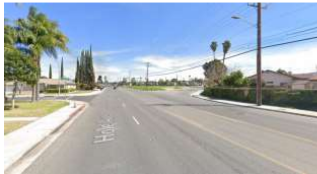
Hole Ave - Wells Ave to Tyler St (Buffered Bike Lane)
