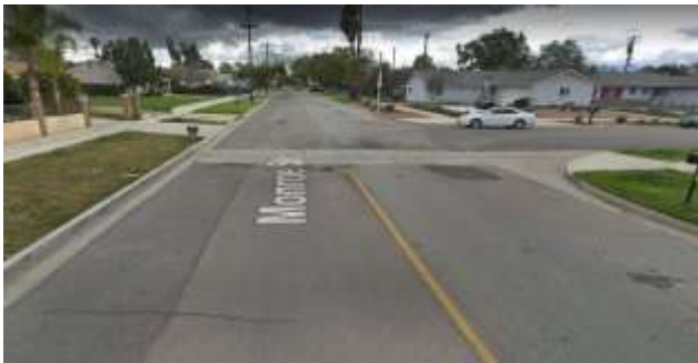
Monroe St - California St to Arlington Ave (Bike Boulevard)
